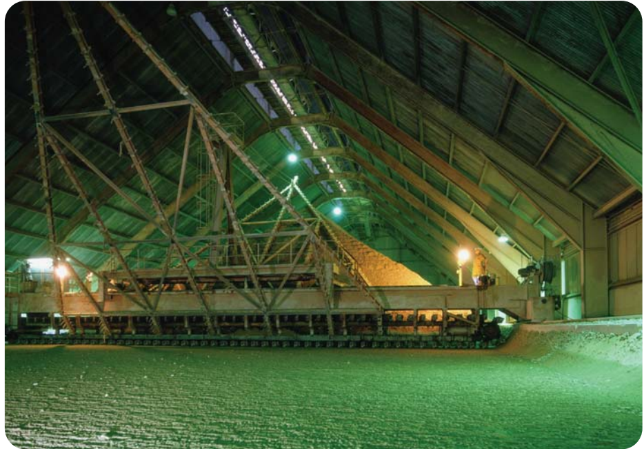
Clay/Limestone Store showing stacker and reclaimer. Max. capacity 43000 tonnes, rail dia. 88m.
